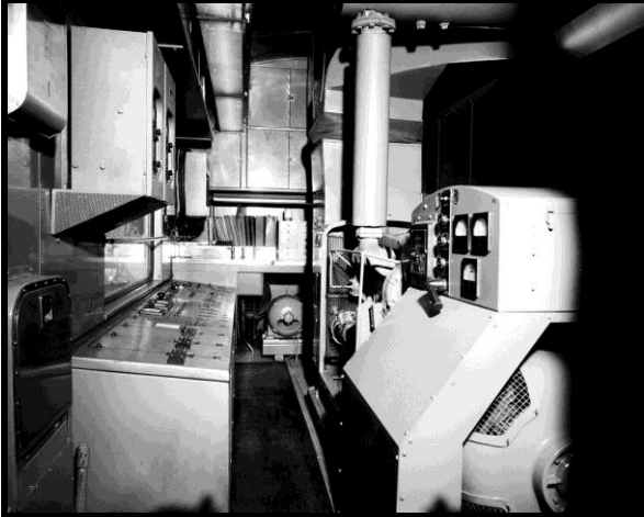
The generator room
