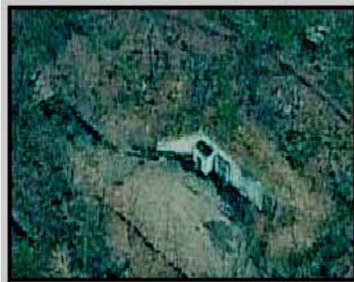
Main Entrance and Parking Lot (Outer Blast Door)
